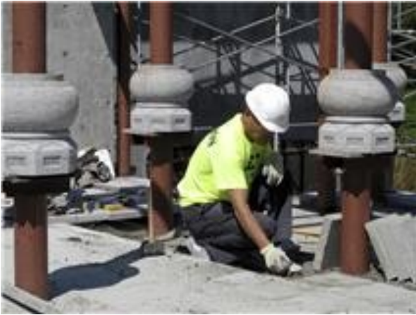
Paving the courtyard
